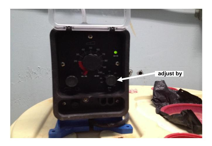
Actual frequency of the metering pump: 60-75 Chlorine consumption: 2 liters per 10 days.
