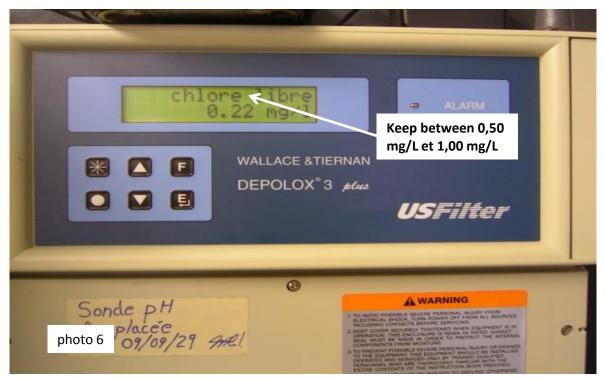
To adjust the chlorine concentration, increase the speed of the chlorine pump (photo 7) if the concentration is too low and decrease if too high. Make small adjustments (around 5 %). It takes at least 12 hours for the adjustment to take effect, so make one adjustment per day
